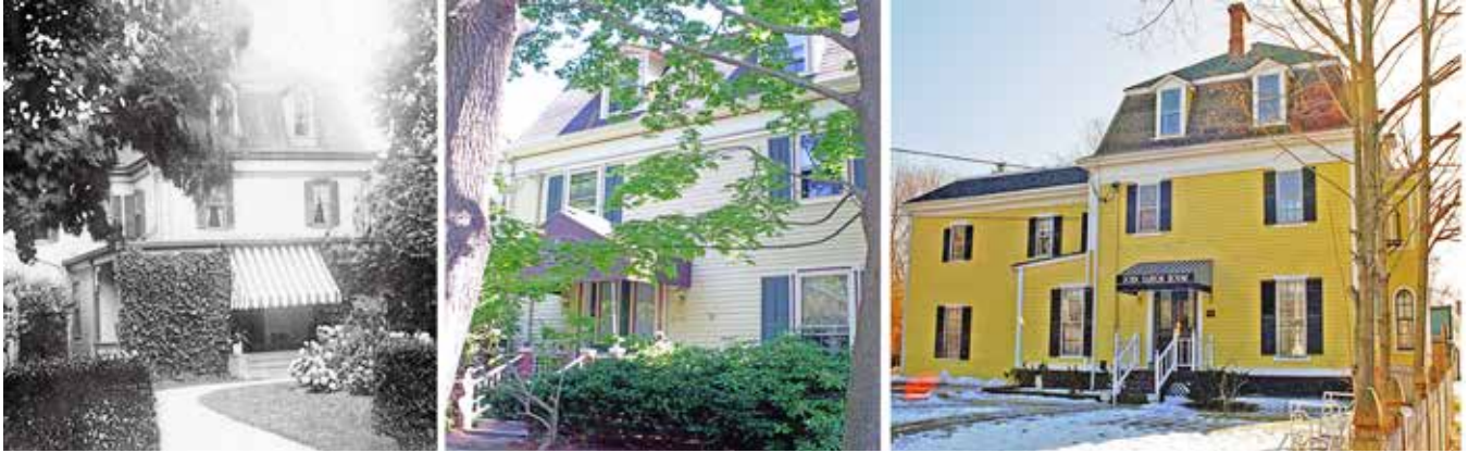
The John Easton House at 23 Catherine Street, Newport, RI was the Charles M. Cottrell home in the early 20th century. At left, a Cottrell family snapshot of the house as it looked in about 1915, with striped awnings and before a later addition was added. At right, more contemporary views showing the addition.
